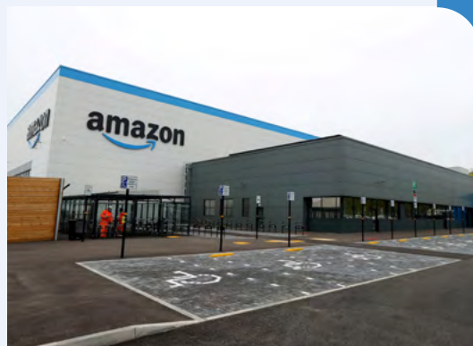
Amazon warehouse, Coventry, West Midlands, UK
